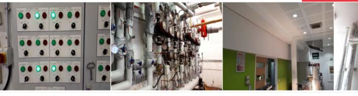
Works included a new building services installation. The lighting system to the main corridor was replaced with modifications to the existing fire alarm system, suspended ceilings were installed and redecoration undertaken.
